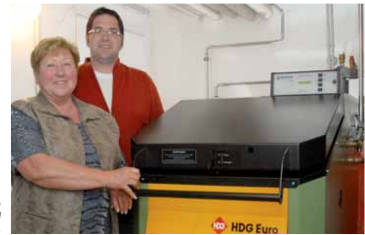
The Schuder family heats with an HDG Euro with 40 kW and 3000 l accumulator.
