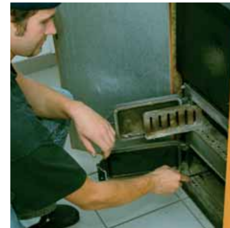
Shake and done! The grate of the HDG SL enables easy ash removal.
